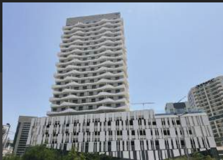
Al Marina Tower, Qatar
